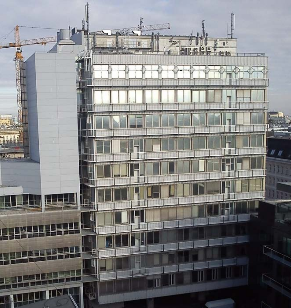
...before the refurbishment Usage: mainly laboratories
