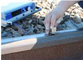
I Railway track superstructure
