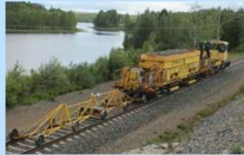
II Railway track embankment
